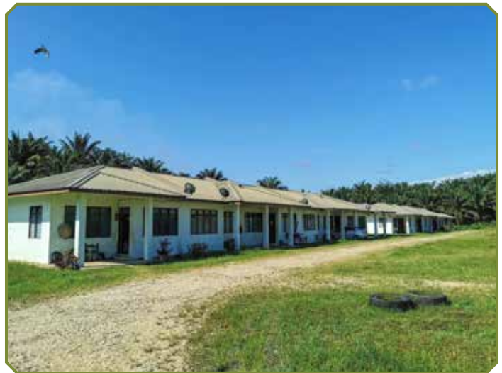
Modern housing quarters built at Sabaju Palm Oil Mill
